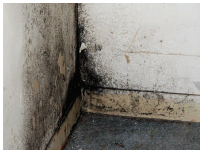
Mold can grow on painted surfaces and other areas where the proper moisture and temperature conditions exist. Photo courtesy of Zinsser.
