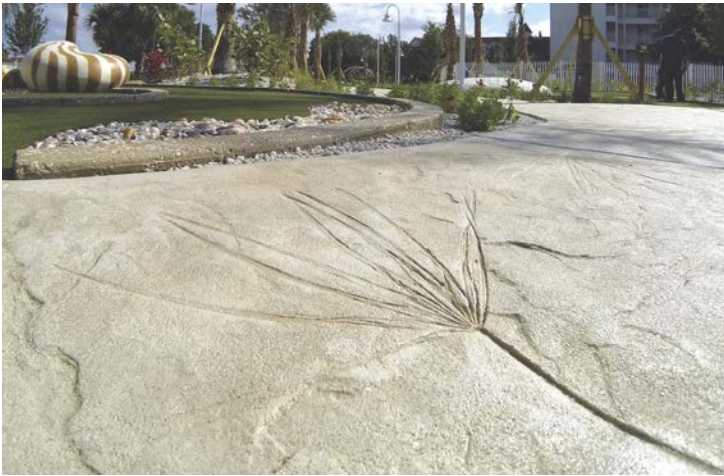
Palm fronds and other native Florida plants were embedded into this decorative concrete walkway during the stamping process, then later removed, to create these fossil-like imprints. Photo courtesy of Edwards Concrete.
