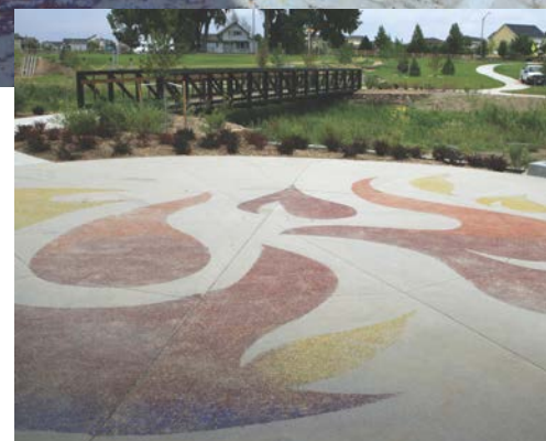
(Top) Concrete artisans hand-seed and trowel blue, red, orange and yellow tumbled glass into concrete. (Lower) A year after installation, the hand-installed flame design of tumbled glass embedded in concrete at Fort Collins’ Radiant Park shows little evidence of wear, other than the dust of foot traffic. Photos courtesy of Colorado Hardscapes.
