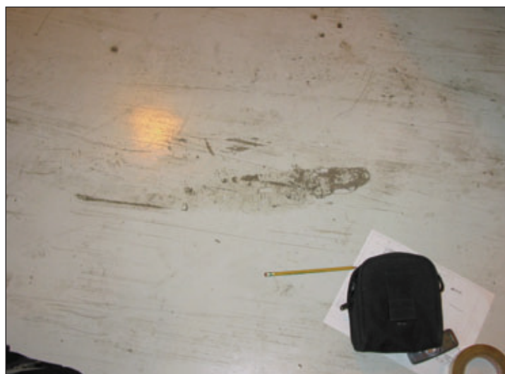
Fig 1: Most scratches on warehouse floor were parallel to length of aisle. Photos courtesy of the author
