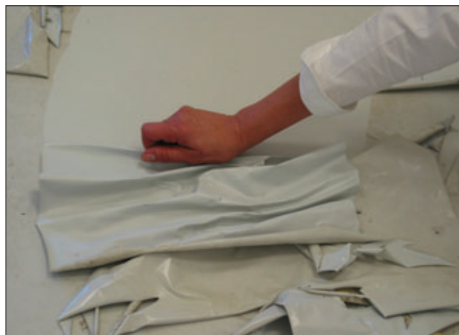
Fig 3: Large sections of coating delaminated with minimal manipulation.
