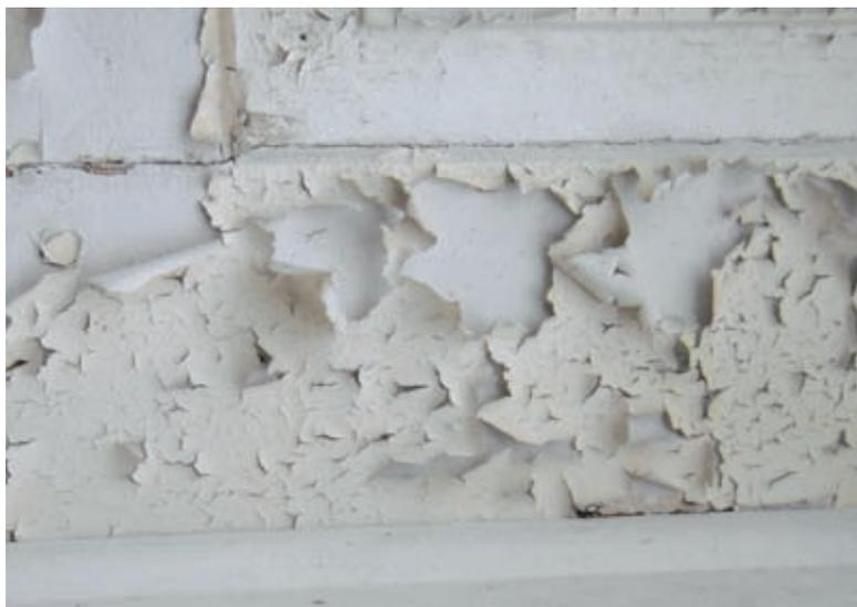
*Excessive moisture in the wood and a degraded wood surface are two primary contributors to coating failure. Photo courtesy Duffy Hoffman, Preservation Specialist.*
