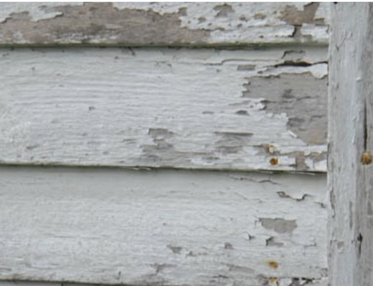
*If coating failure is apparent, all poorly adhered coating and the degraded wood layer must be removed prior to application of new paint or coating.
