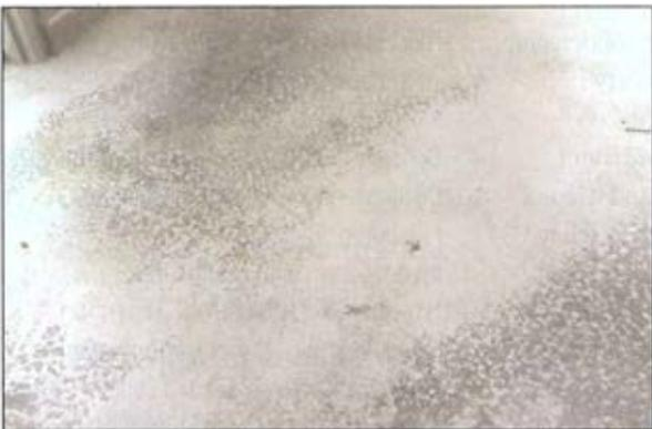
**Fig. 2:** Laitance, a thin, weak layer of fines and cement residue, is related to unreacted concrete constituents.
