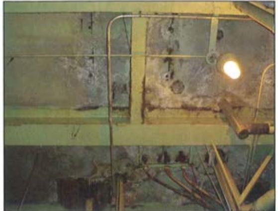
**Fig. 3:** If the source of moisture that causes efflorescence is not eliminated, freeze/thaw cycling or other moisture-related effects can weaken the substrate.
