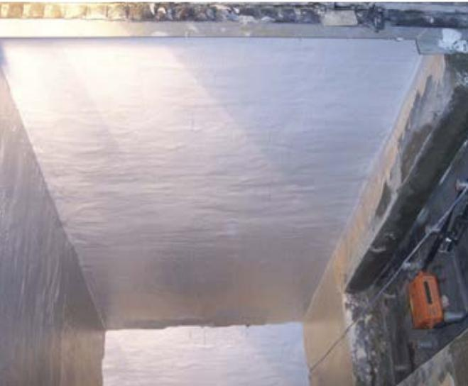
For the new lining to perform properly, surface preparation must meet acceptance criteria such as those described in the SSPC/ NACE joint standard on preparing concrete for coating.
