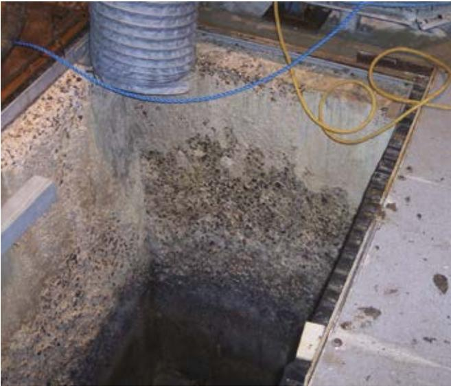
*Properly specifying the repair of deteriorated concrete, like the interior walls of this wastewater collection basin, depends on taking into account many more contaminants and conditions than the boilerplate phrase, “clean and dry,” accounts for.*
