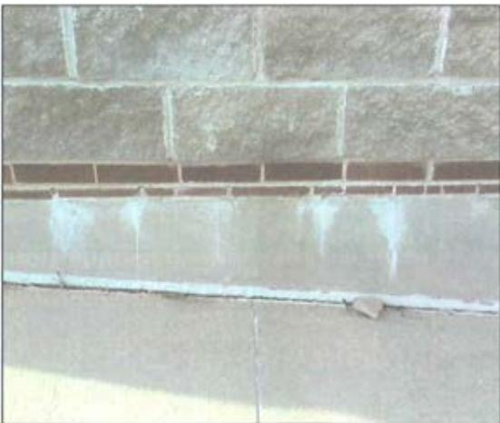
*Fig. 1: Efflorescence has a granular or powdery appearance. The effect is caused by moisture vapor transmission. Photos courtesy of the author.*
