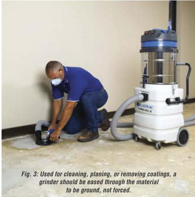
*Fig. 3: Used for cleaning, planing, or removing coatings, a grinder should be eased through the material to be ground, not forced.*
