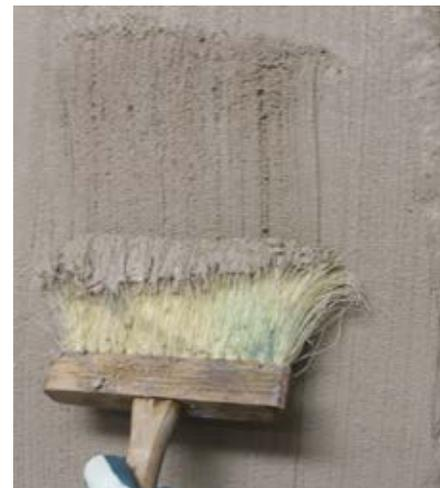
Fig. 1: Typical broom-finished surface
