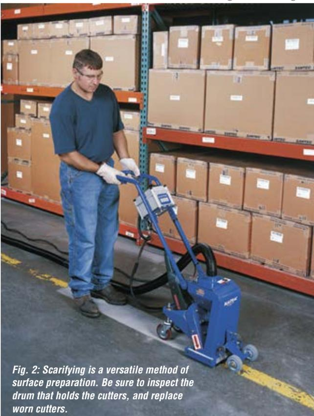
*Fig. 2: Scarifying is a versatile method of surface preparation. Be sure to inspect the drum that holds the cutters, and replace worn cutters.*
